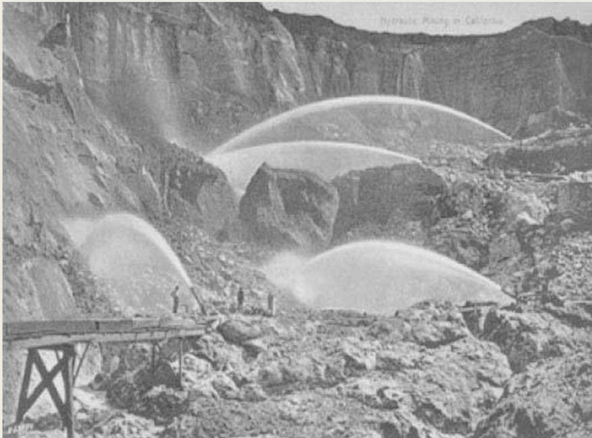
**Hydraulic mining, or hydraulicking, is a form of mining that uses high-pressure jets of water to dislodge rock material or move sediment. In the placer mining the resulting water-sediment slurry is directed through sluice boxes to remove the gold.**
