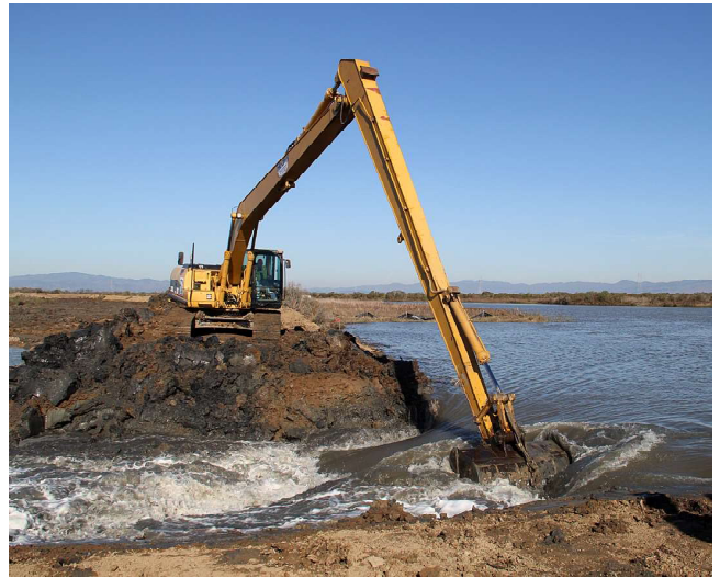
Cullinan Ranch levee breach, January 6, 2015
