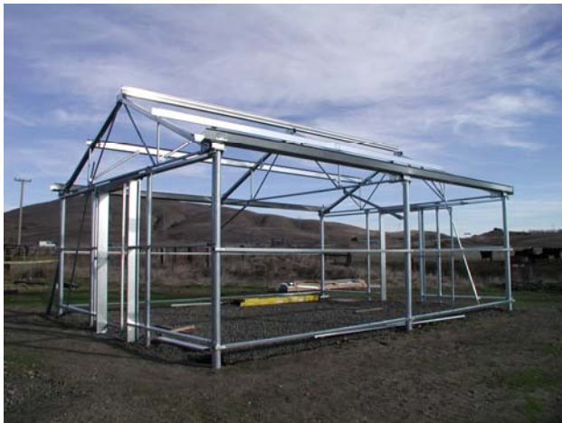
Construction of the greenhouse.
